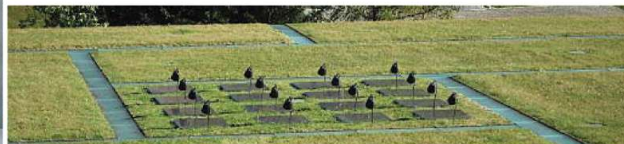
GreenRoof System by ZinCo, Germany downlight in the skylight area
